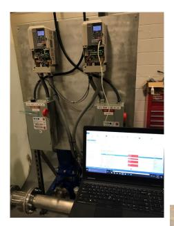
OPSCO provides pump and control field diagnostics and troubleshooting support. Our factory trained salespeople offer pump and control start-up support. We also provide onsite motor testing with our Baker ST-103 Winding Analyzer.
